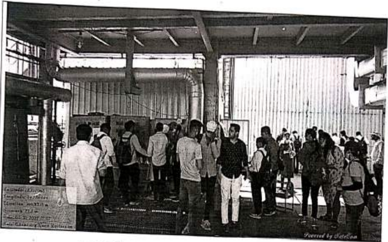
Students Collecting Information on Boiler Process for Steam Generation
